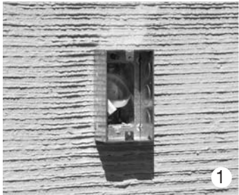
1 Attach UL-listed extension box to pre-wired and mounted electrical box.
