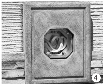
4 Complete placement of Cultured Stone® veneer or other exterior material around Electrical Box Stone.
