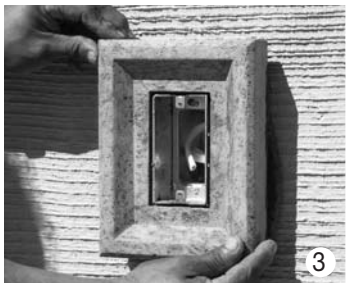
3 Center Electrical Box Stone over the extension box. Level and plumb. Use removable shims if required.
