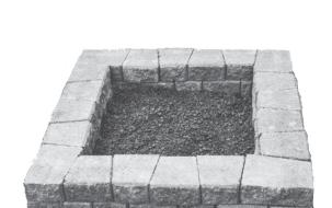
**3.** Transfer the second layer. Note the 11-inch side of the corner block will now be over the 6.5" side of the corner block beneath.
